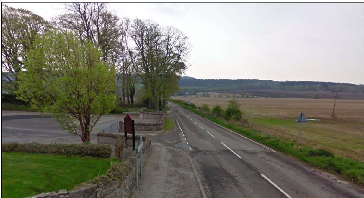
Figure 39: Photo showing the end of existing footpath at the church
