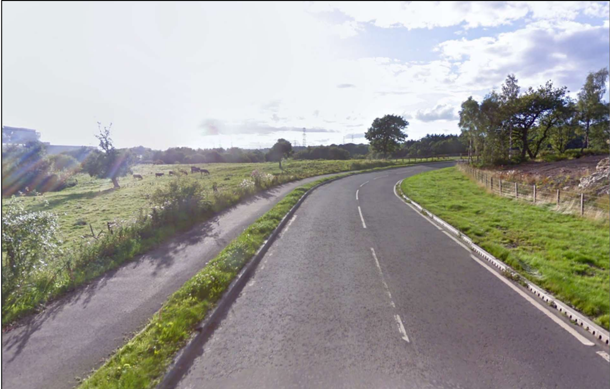
Figure 21: Example of a shared use path
